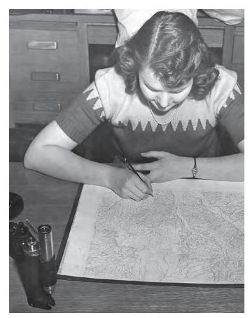
**Figure 23.** Pen-and-ink drafting for map production was used from the early 1940s through the mid-1950s. Inking contours by hand required a light touch to maintain consistent line weight (1952).
