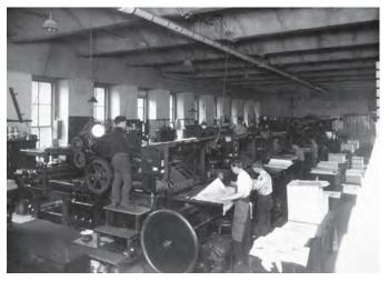
**Figure 9.** U.S. Geological Survey printing presses for use of lithostones in printing topographic maps.
