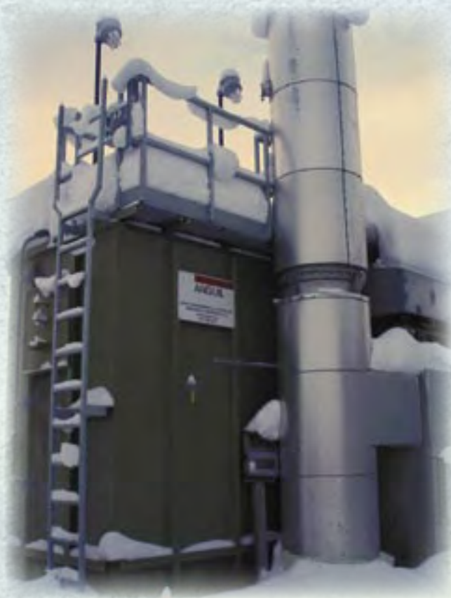
This Anguil incinerator burns vapors collected during the ballast water treatment process. Two such units have been installed at the Ballast Water Treatment Facility. Photo by Tom Kuckertz.
