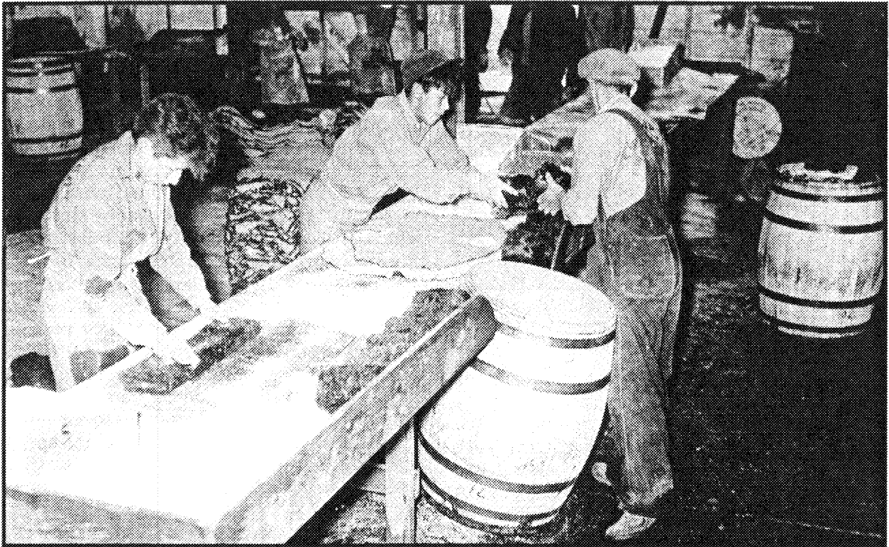
Figure 27. When the skins were dry, they were bundled in salt or borax and packed in barrels -- note man packing with his feet at right.
