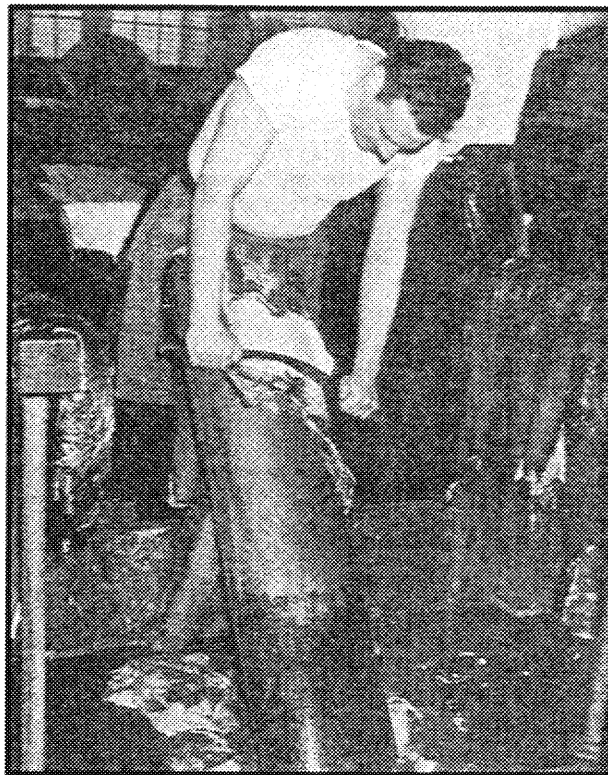
Figure 22. From the wash tanks the skins went to a blubbering beam like this one shown at St. Paul, and the blubber was removed with double-handled knives.
