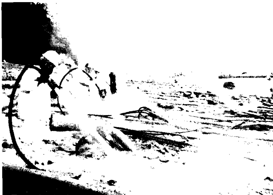
Workers washed oil with hot-water hoses toward the water where skimmers picked up the oil.
