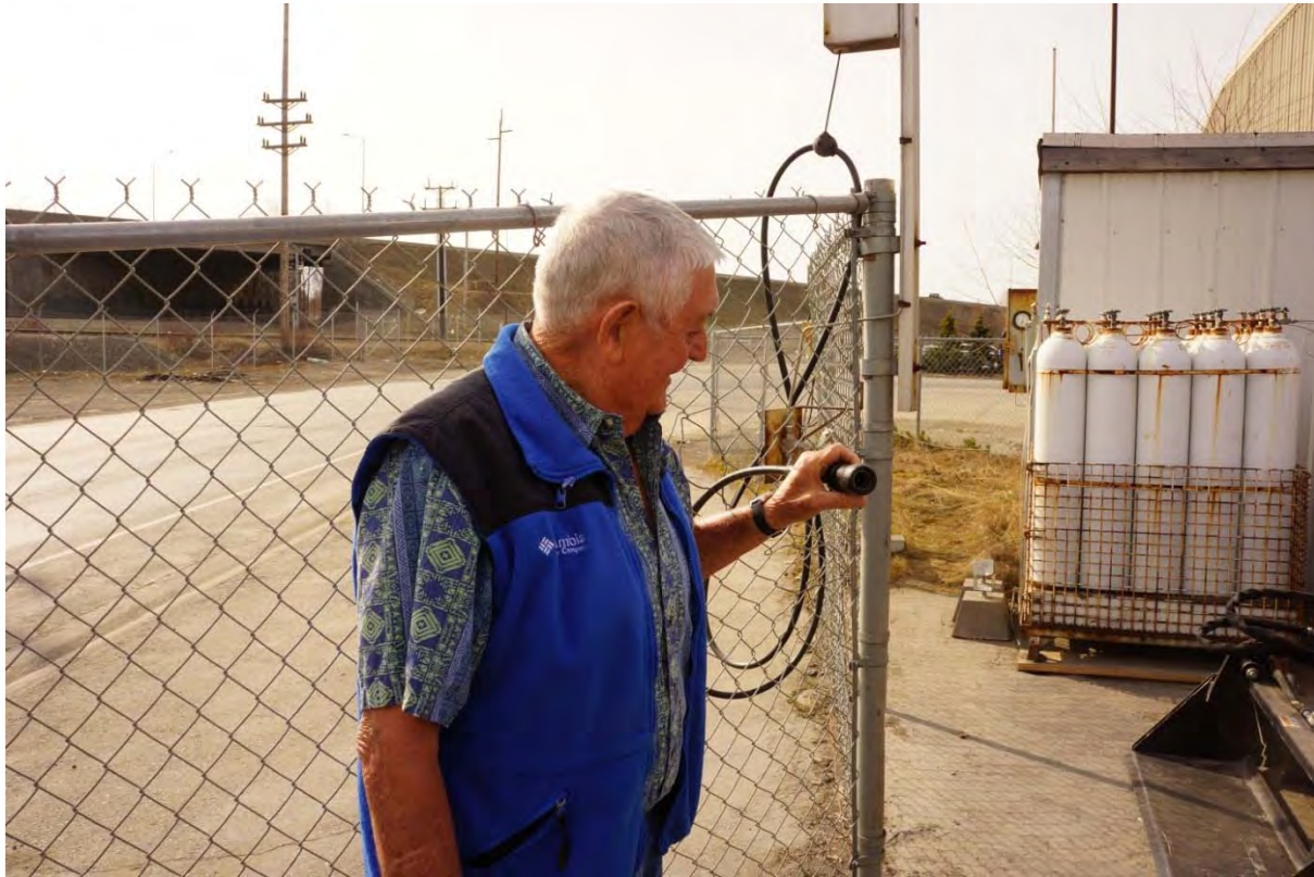
Figure 12. CNG Fueling Hose, with Storage Tanks, Anchorage, Ditch Witch.
