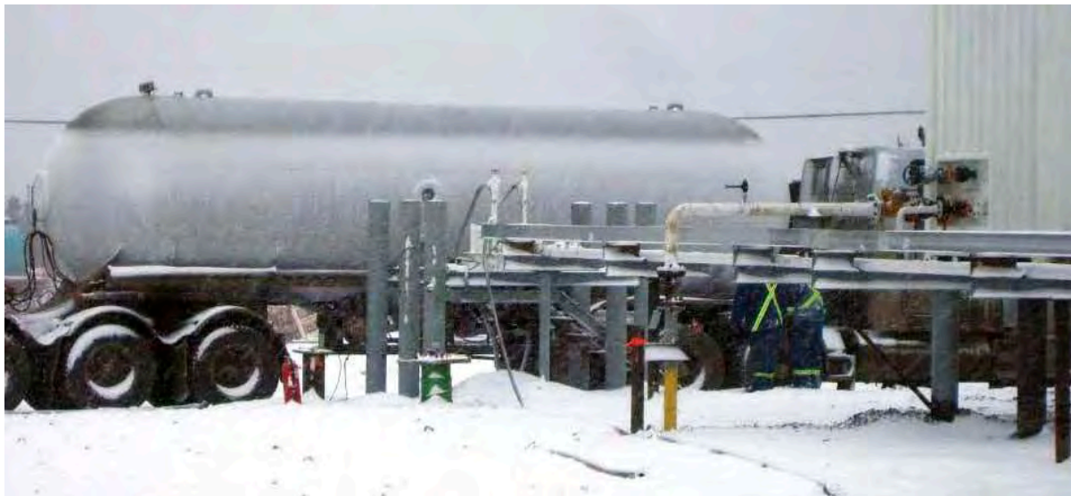
Figure 11. LPG Feed Tanks and Vaporizing Unit, Nunavut, Northwest Territories, Canada.
