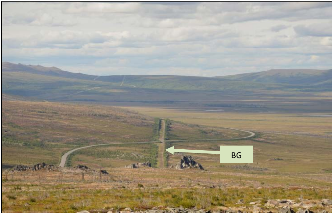
South of Pipeline Milepost 300, but still in tundra, the Dalton Highway curves, and the pipeline runs in a straight line underground (Image source: Center for Land Use and Interpretation; http://clui.org/page/trans-alaska-pipeline-0 )
