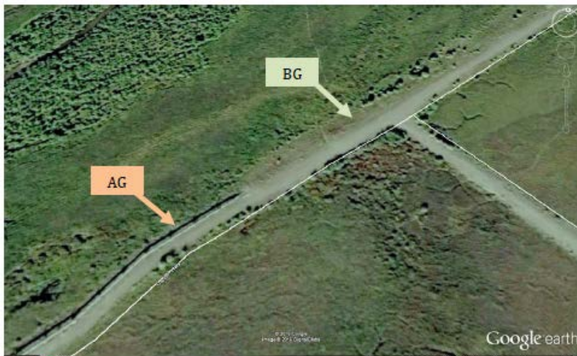
Aerial View of Belowground Sections of TAPS on Alaska's North Slope
