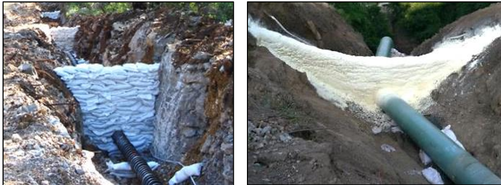
Figure 5. Ditch Plugs Made from Different Types of Materials
