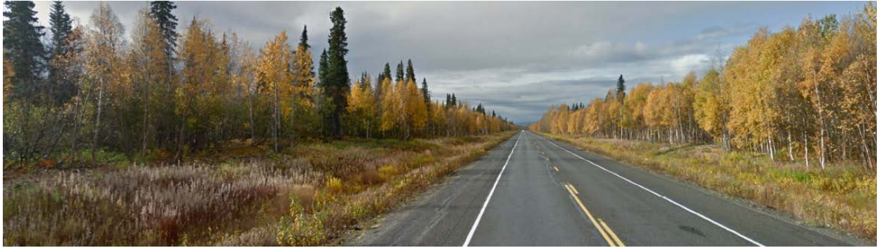
a. Existing Conditions
