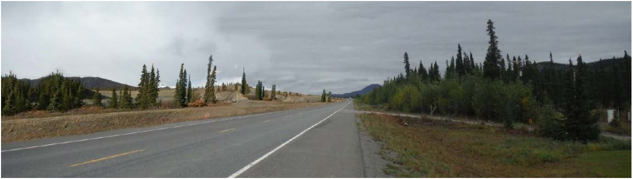
b. After Construction
