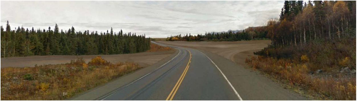
b. After Construction
