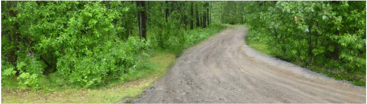
b. After Construction
