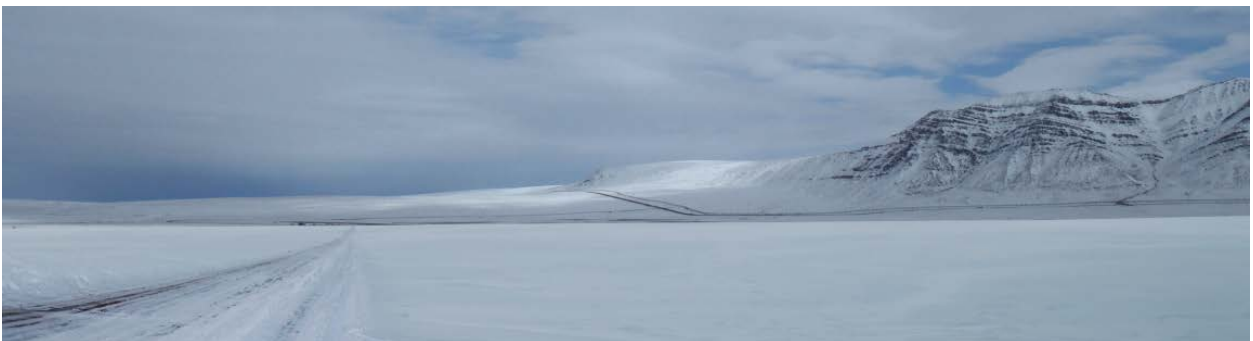
f. Winter Conditions After Constructions
