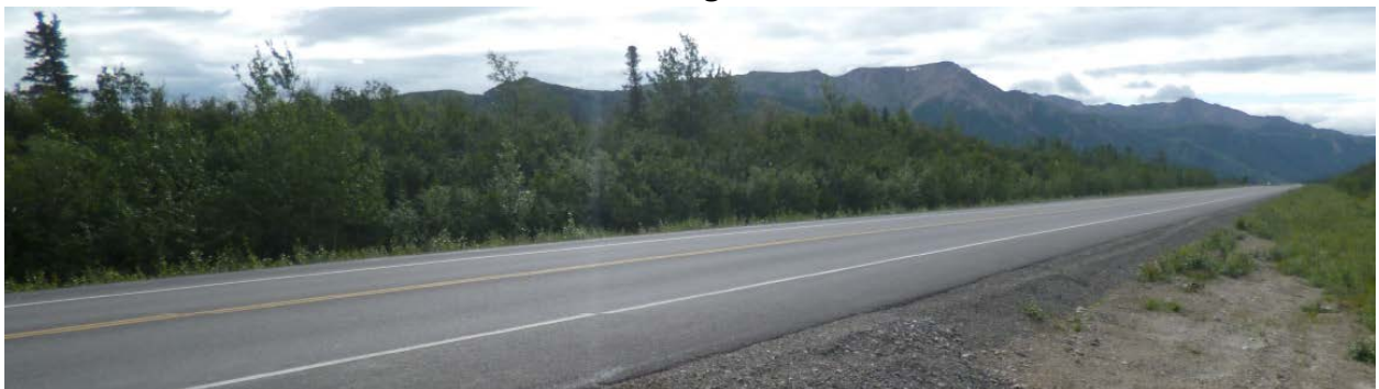
a. Existing Conditions
