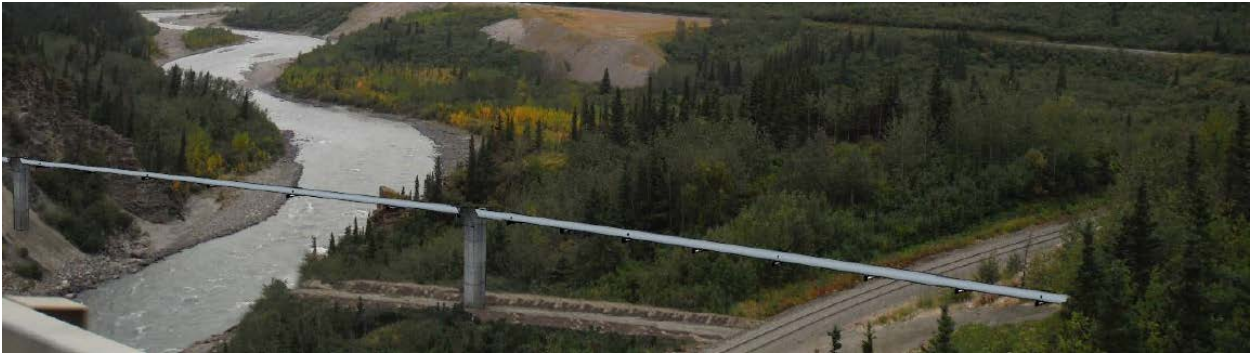
b. After Construction
