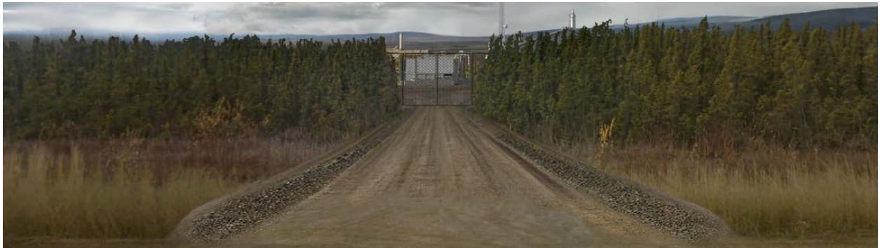
b. After Construction
