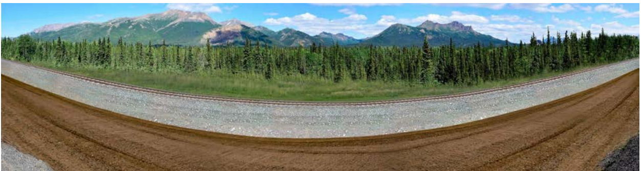
b. After Construction
