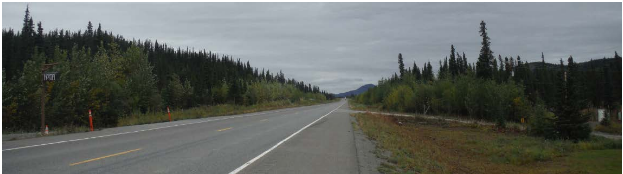
a. Existing Conditions
