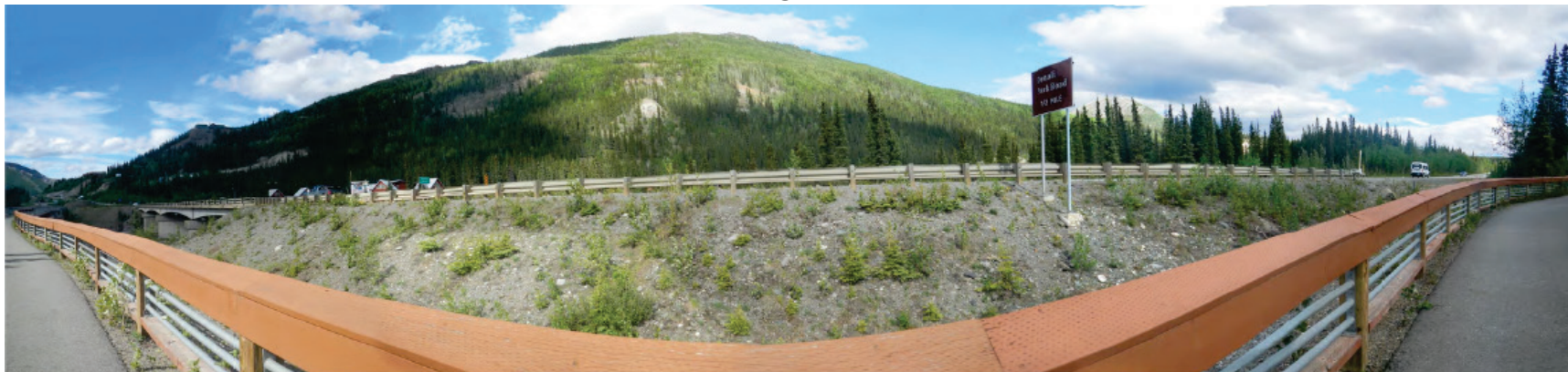
Figure E.1.7-1: KOP 2018-13: Nenana River Pedestrian Bridge; View of the Denali Avoidance Alternative to the South
