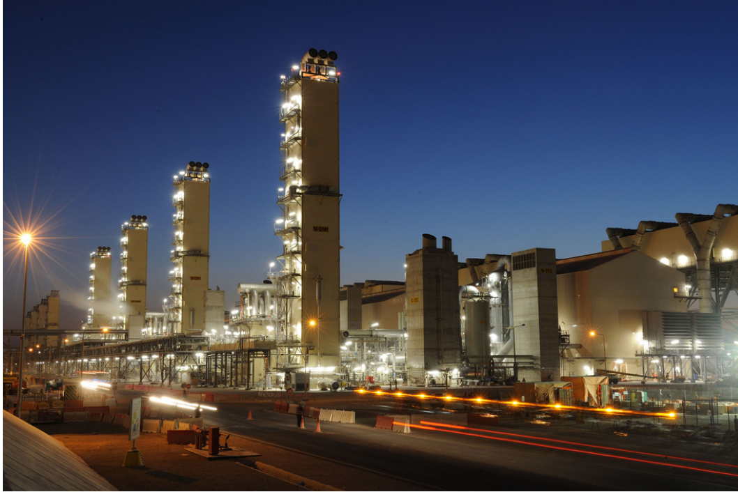
Source: Shell Air separation towers at Shell's Pearl GTL plant in Qatar.
