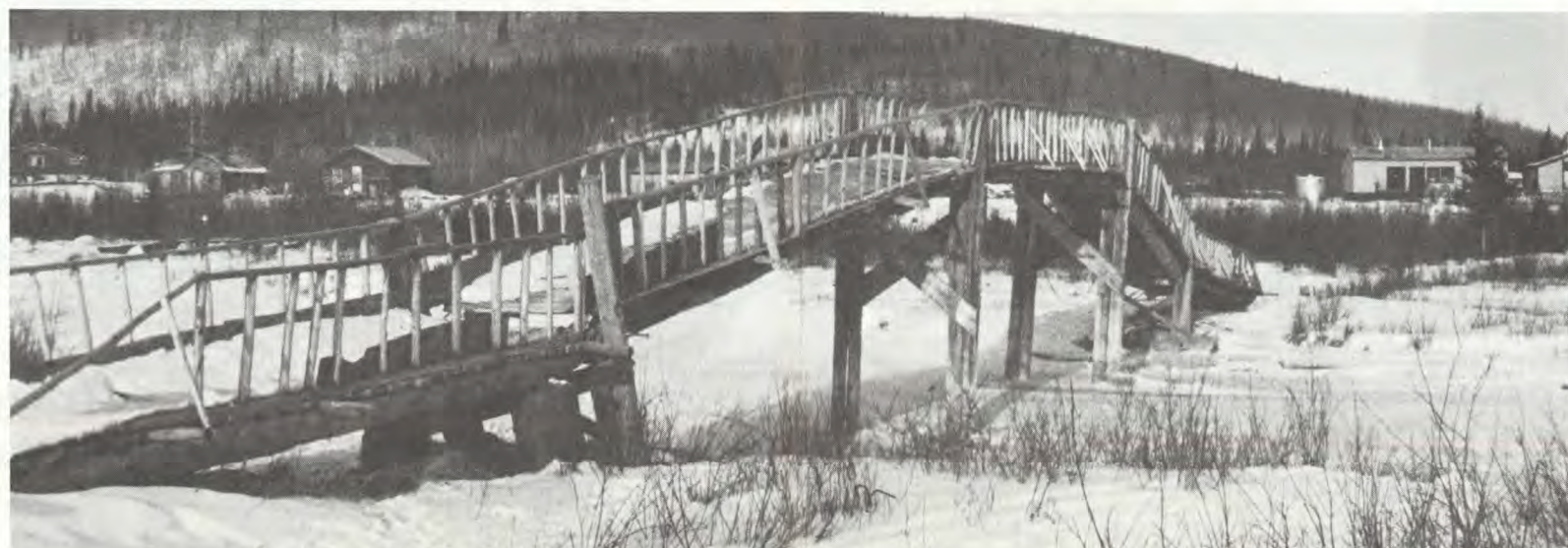
The footbridge which leads from the airstrip across the Tetlin River to the village has been damaged due to frost heaves.
