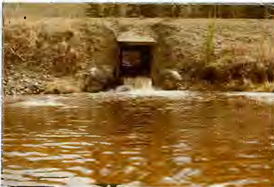
5/11/81 - Unnamed Creek (RX 106-3) looking upstream at Alaska highway culvert outlet.
