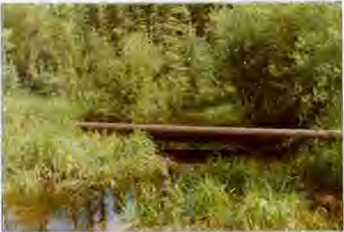
7/9/81 - Unnamed Creek (RX 119-2) looking upstream at Haines pipeline crossing.
