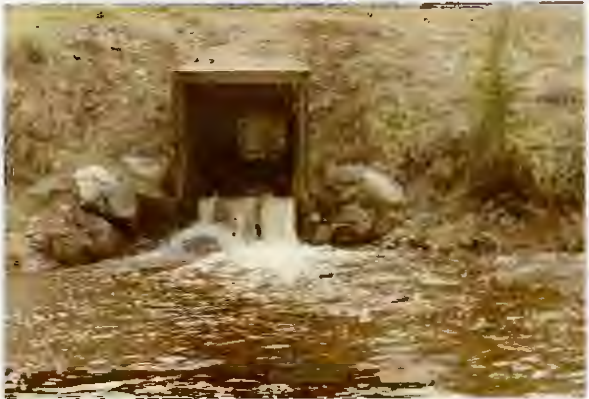
5/26/81 - Unnamed Creek (RX 106-3) looking upstream at Alaska highway culvert outlet.
