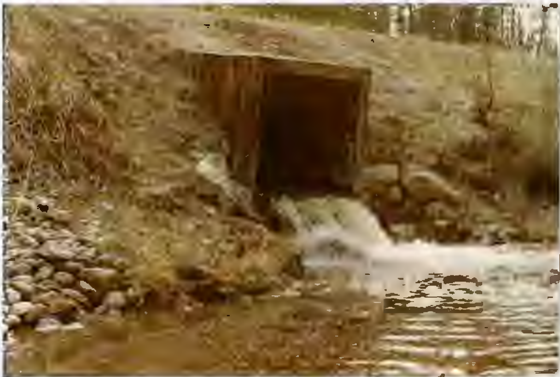
5/26/81 - Unnamed Creek (RX 106-3) looking across Alaska highway culvert outlet.
