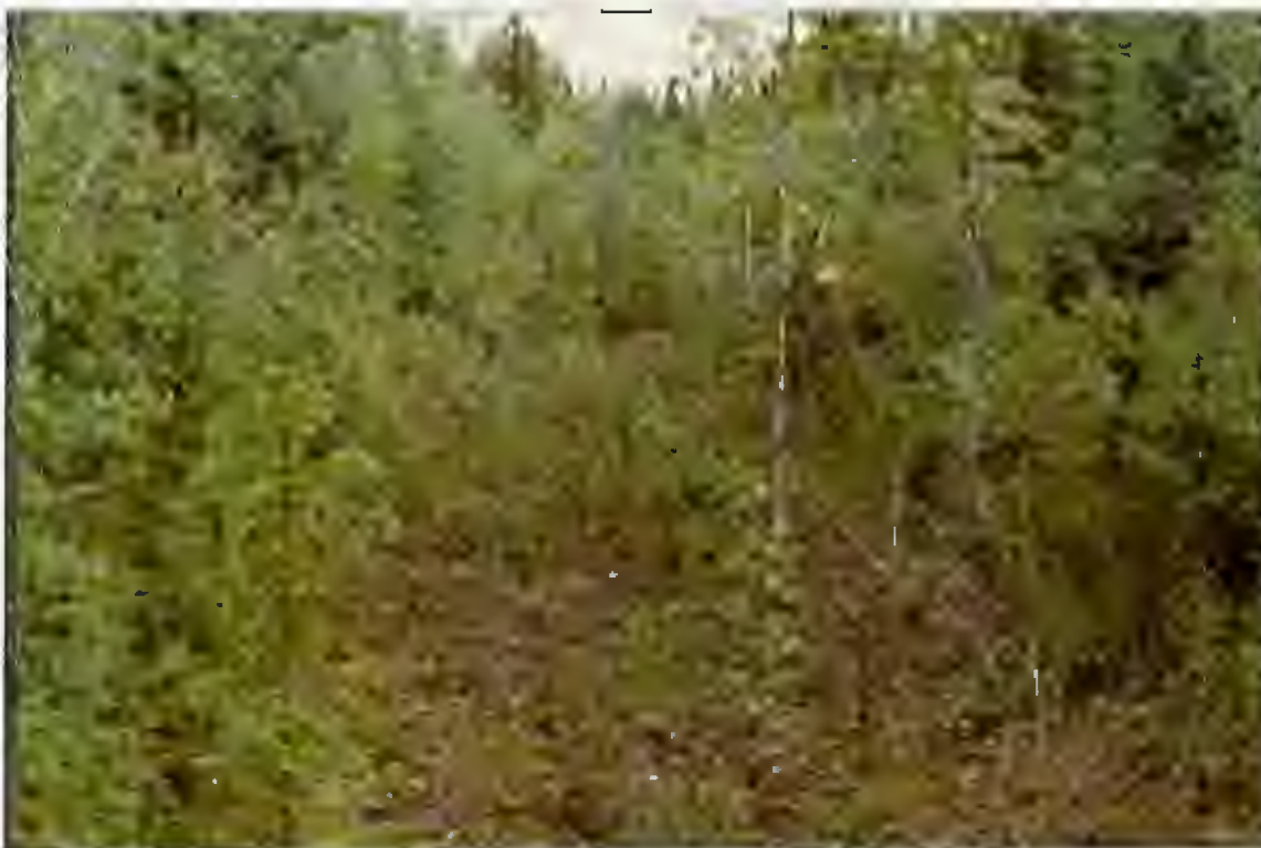
7/17/81 - Granite Creek? (RX 099-1) looking downstream from Haines pipeline right-of-way. Bulldozer clearing continued.
