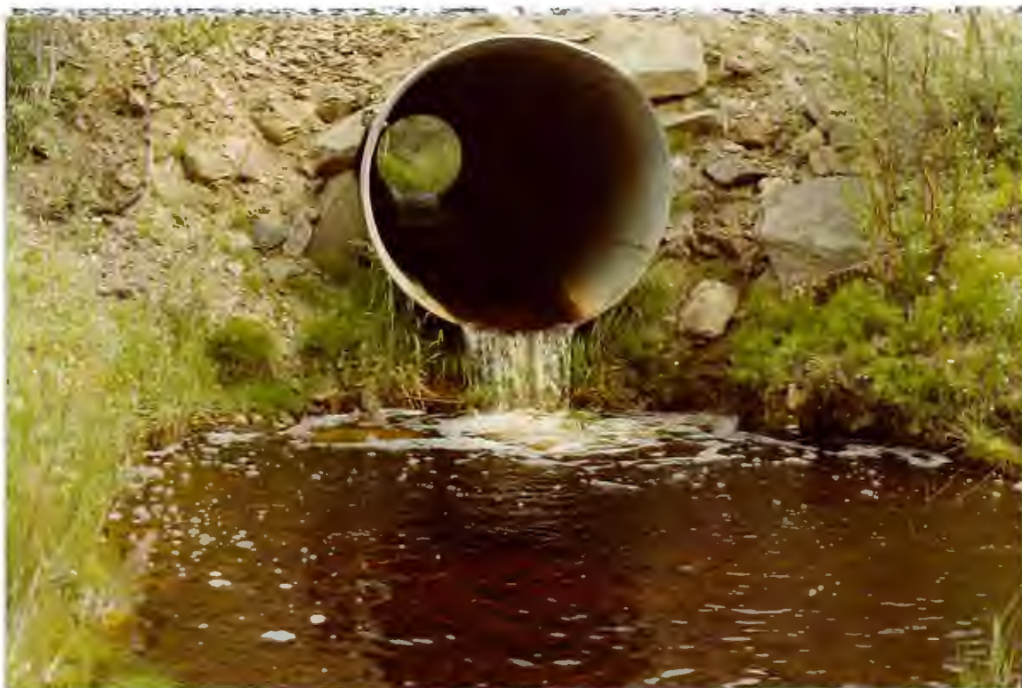
8/6/81 - Unnamed Creek (RX 123-1) looking upstream to Alaska highway CMP.
