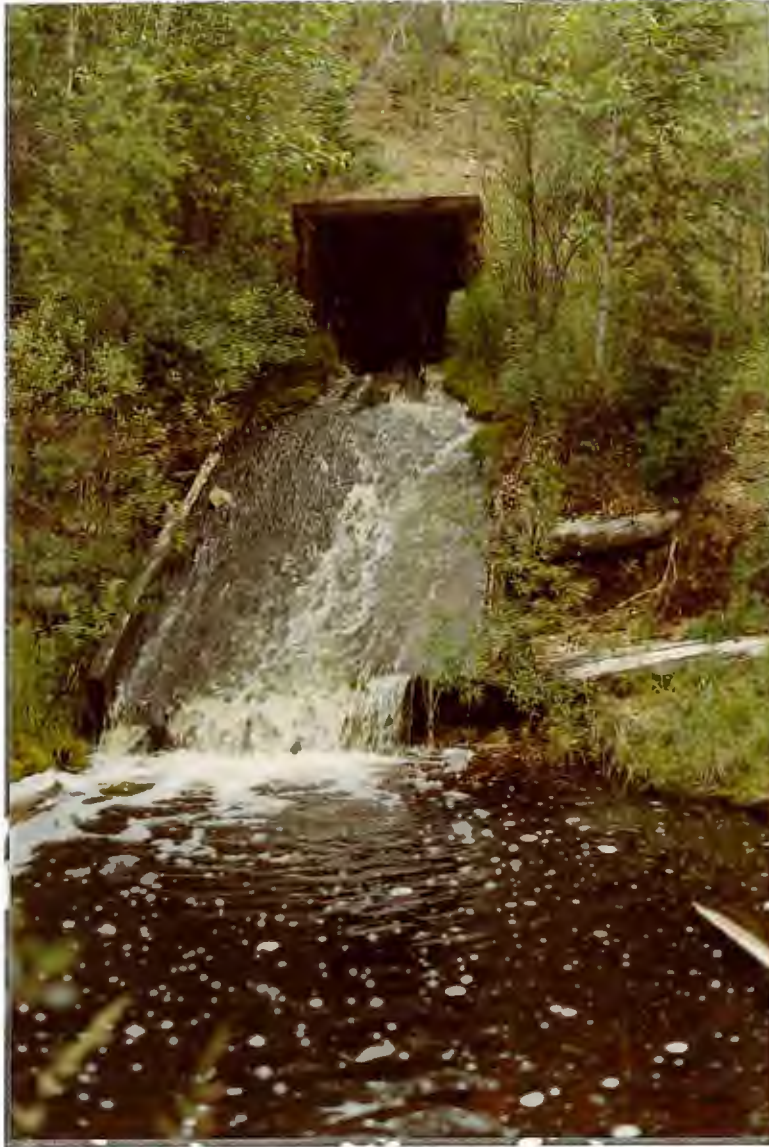
8/6/81 - Lethe Creek (RX 124-2) looking upstream to Alaska highway culvert outlet.
