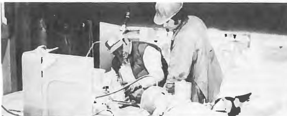
**Foothills and contractor personnel monitor testing of high-pressure discharge piping at Richmond compressor station.**
