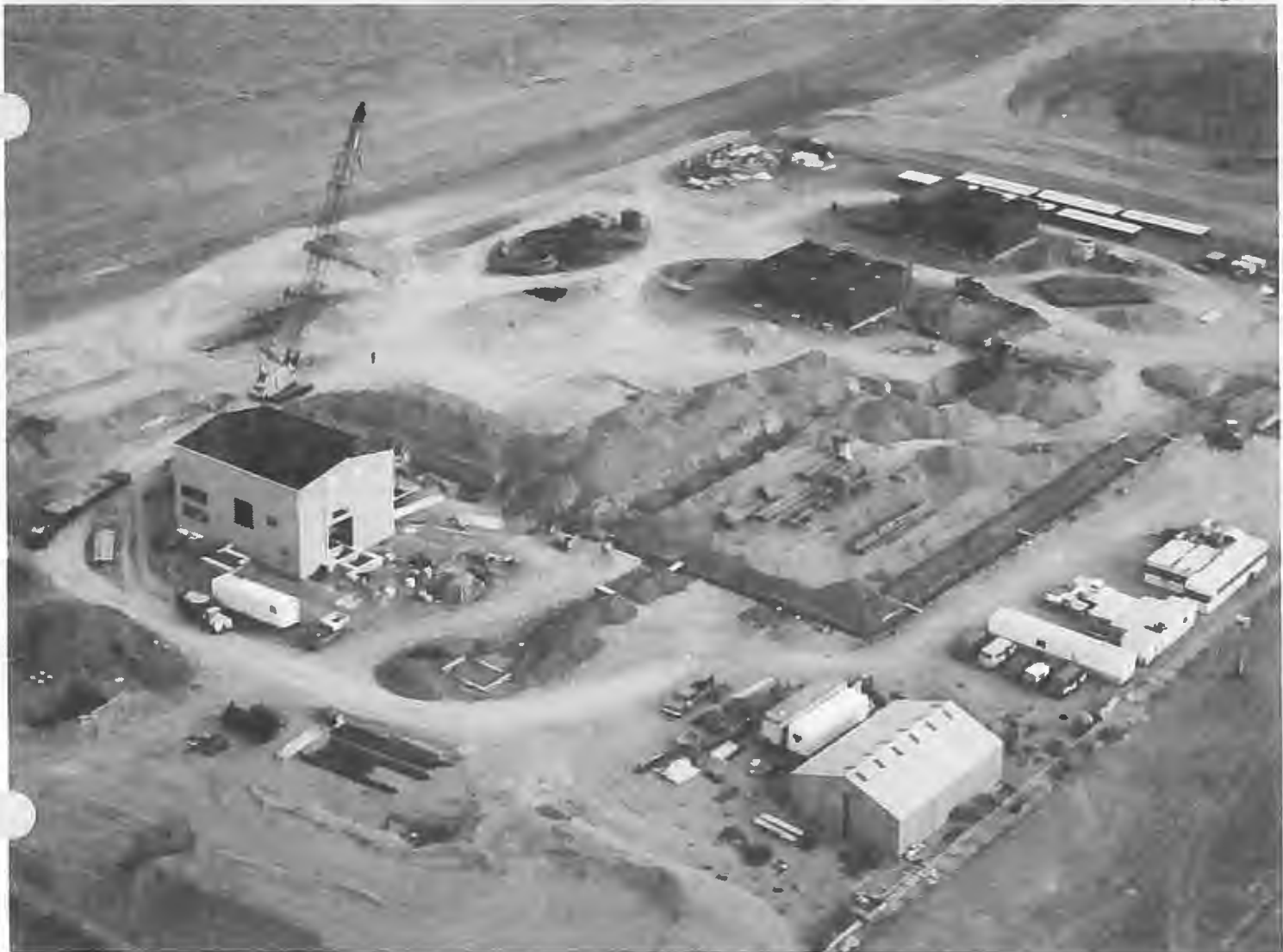
Aerial view of compressor station under construction near Jenner, Alberta.
