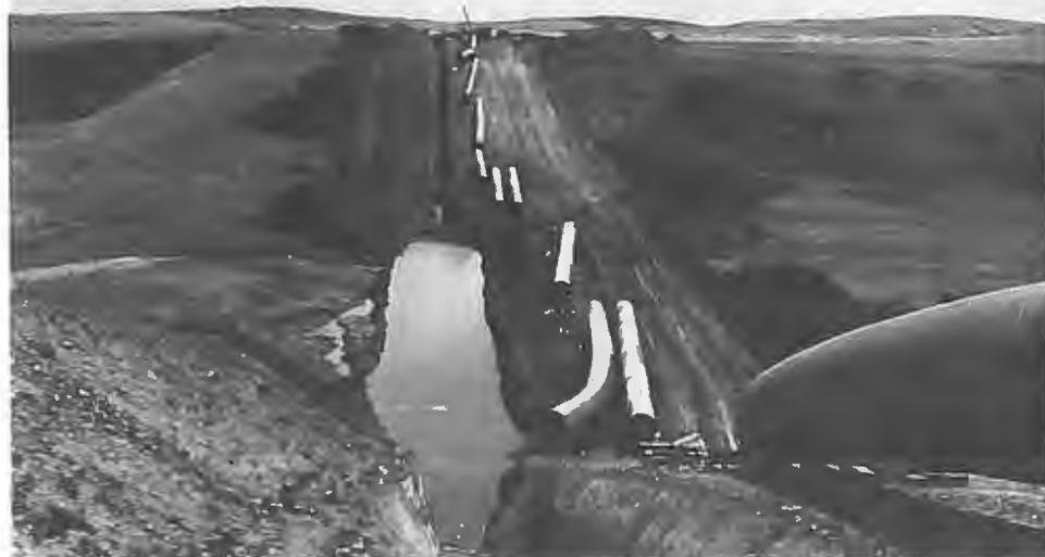
Tie-in to a road crossing east of Jenner (above). Pipe strung along the right-of-way and ditch prepared for crossing Severn Creek near Rosebud (below).
