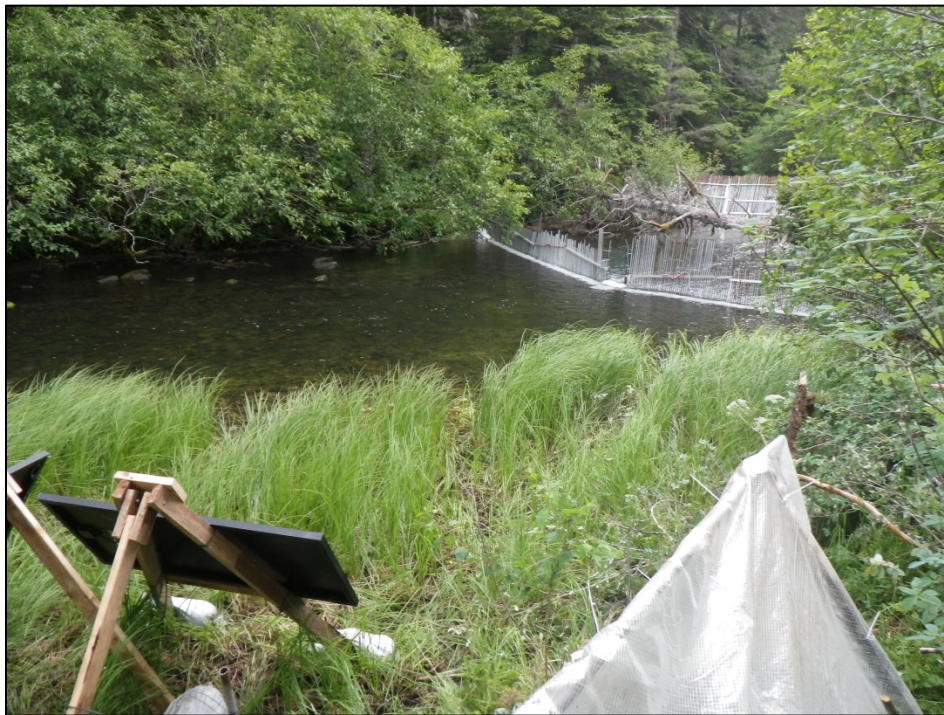
Figure 7.—Lake camera weir, directly below the outlet of Kanalku Lake, 2014. The standard picket weir is visible downstream of fallen tree. (©2014 ADF&G/Photo by Raymond F. Vinzant.)
