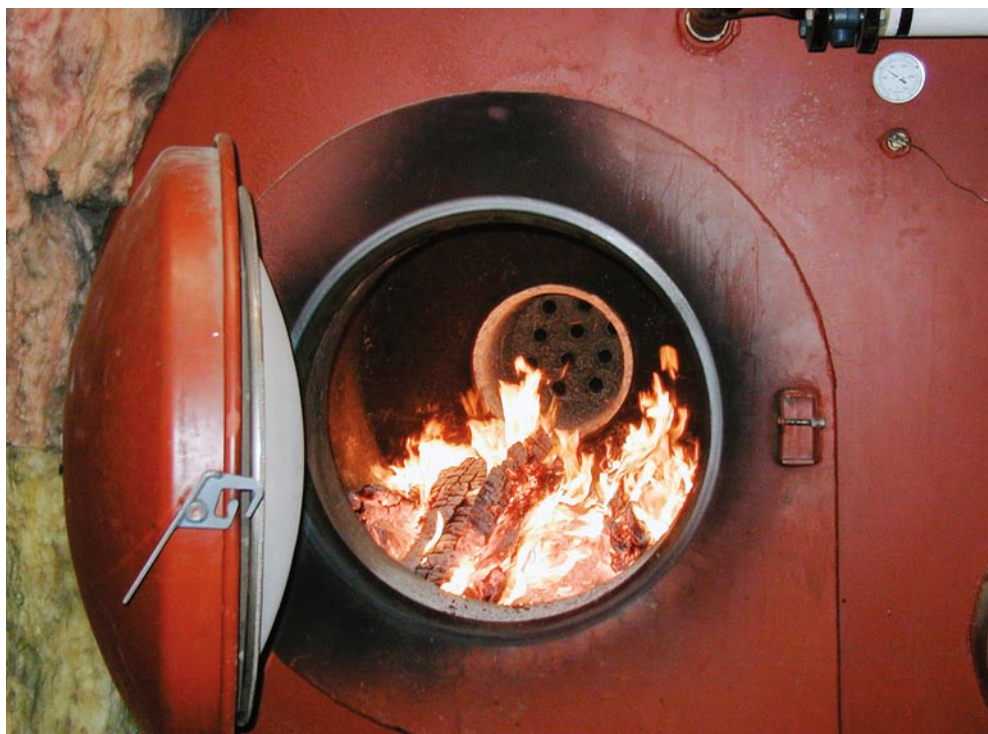
Figure 3—High-efficiency cordwood energy system showing open firebox and burning embers (note that water storage reservoir surrounds firebox).
