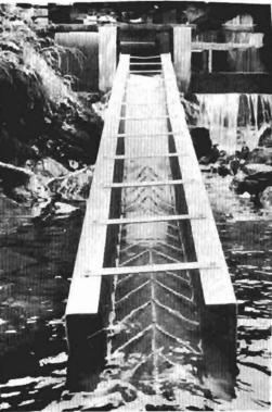
and other materials used in many other states. The term "steep-pass" refers to the need for bypassing falls or dams in as short a horizontal distance as possible, to cut down on labor, materials, and other construction costs.
