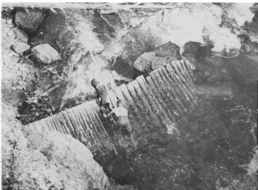
Figure 3. Weir constructed by Department on tributary of Taku River.
