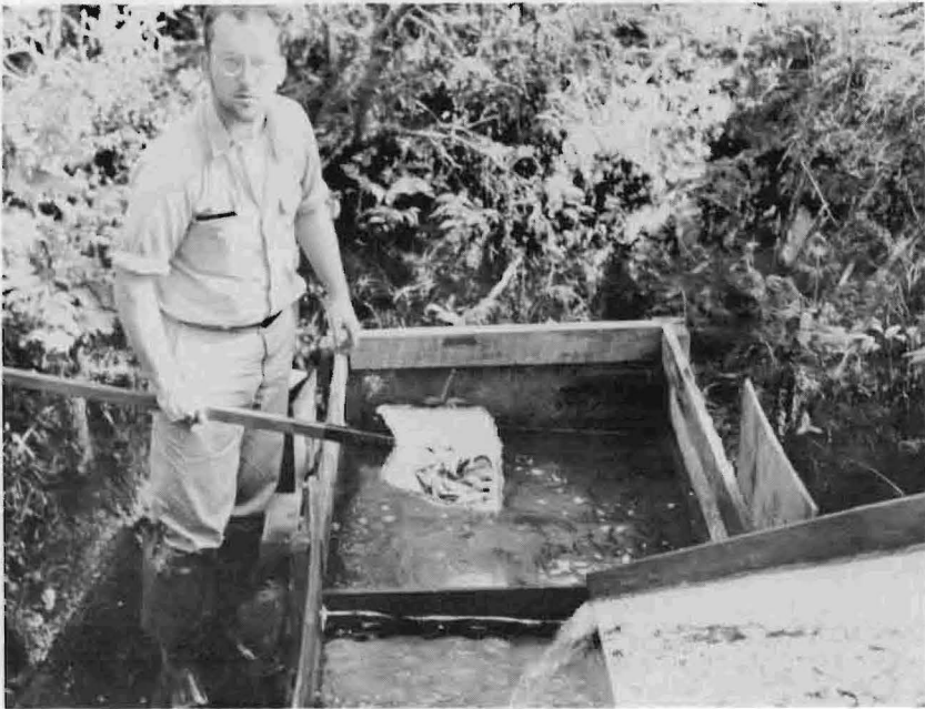
Weir with inclined screen by-passes all red salmon fingerlings leaving Ruth Lake to trap for counting and subsequent release downstream.
