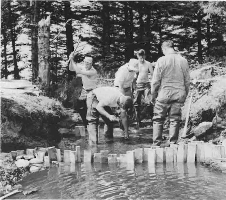
Figure 9. Building a screen structure in the outlet of a lake to prevent the stocked steelhead from migrating out of the lake.
