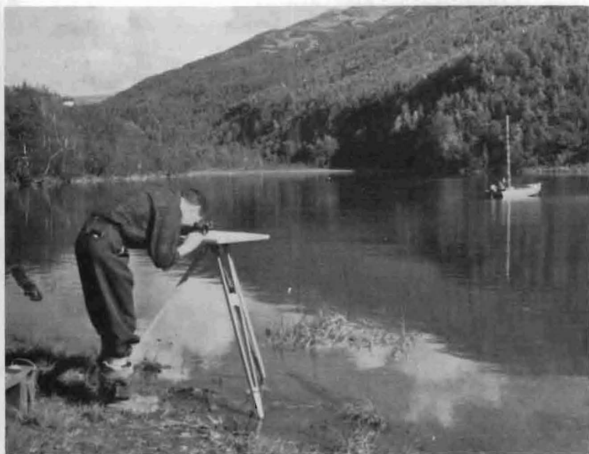
Figure 6. Biologist surveying a lake using an alidade and stadia rod.
