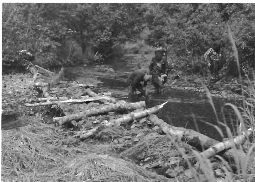
Plate 3. FALLS CREEK DIKE.
