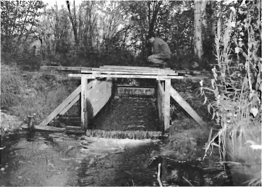
Plate 2. BIRCH LAKE WATER LEVEL CONTROL DAM.
