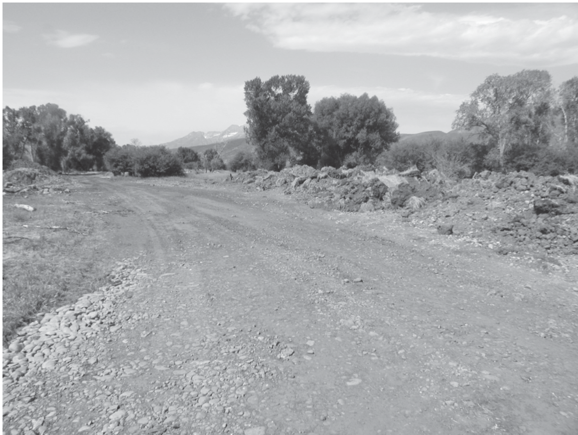
Figure 2 —PRRP haul route. Note that the top foot of soil, which contains plant roots and seeds, has been stockpiled to the right of the road. This minimizes handling of the topsoil. Decommissioning of the route would follow the sequence of removing any road fill, grading to establish proper contour, ripping (if necessary), and replacement of topsoil.
