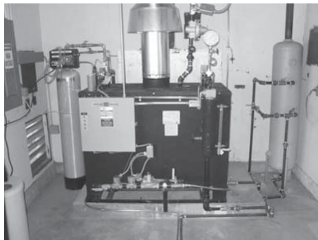
Figure 3 — This propane boiler supplies 160 °F (71 °C) steam to a 24-ft by 47-ft by 10-ft high (7.3-m by 14.3-m by 3-m high) room used to sterilize used Styroblock ™ containers at USDA Forest Service Lucky Peak Nursery, Idaho.
