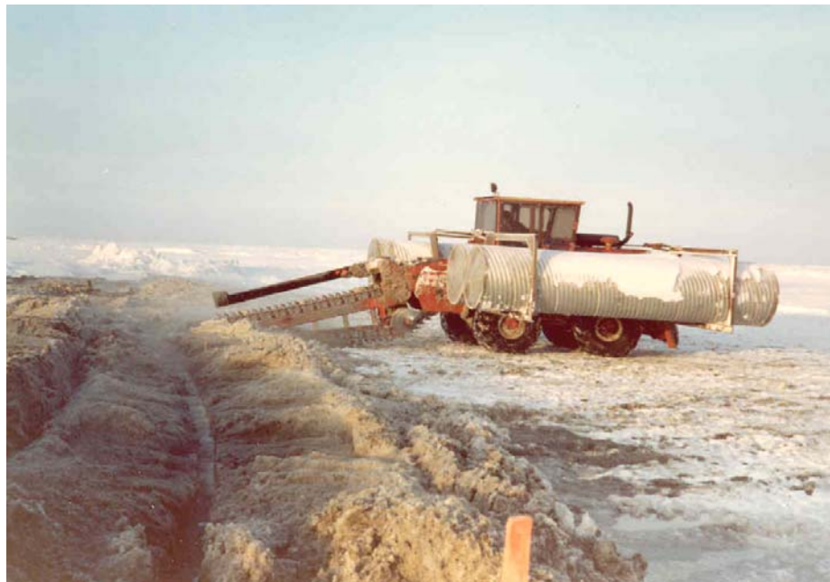
Widening of the ice hole with a Ditchwitch cutting machine (equipped for buoyancy tanks in case of break-in)
