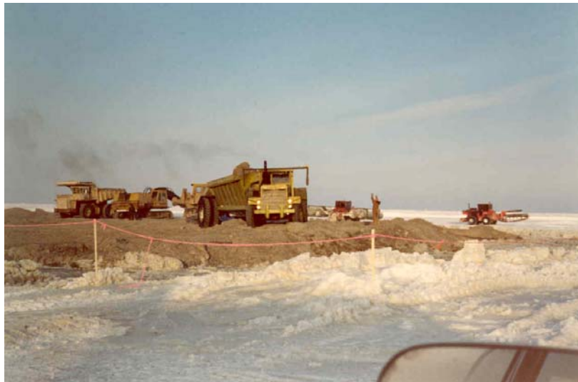
After surfacing of the gravel, trucks drive onto the new island to unload
