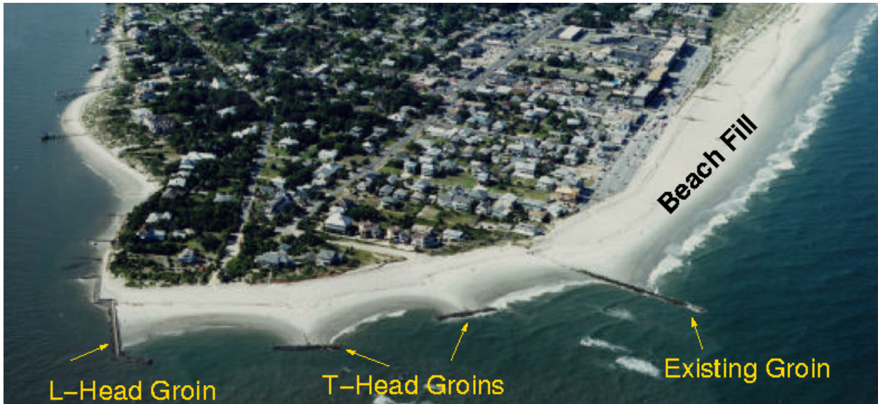
Figure 10. Terminal groin field at Tybee Island, GA (photograph courtesy of Olsen and Associates, Inc.)
