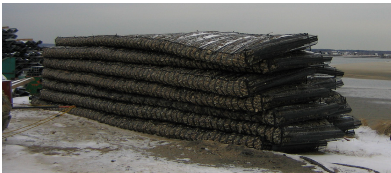
Figure 2. Stack of filled marine mattresses staged for placement on National Shoreline Erosion Control Development and Demonstration Program (Section 227) project in Seabrook, NH (photograph by Kevin Knuuti, CHL)
