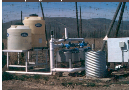
Sand filters and chemical-storage tanks for a drip-irrigation system
