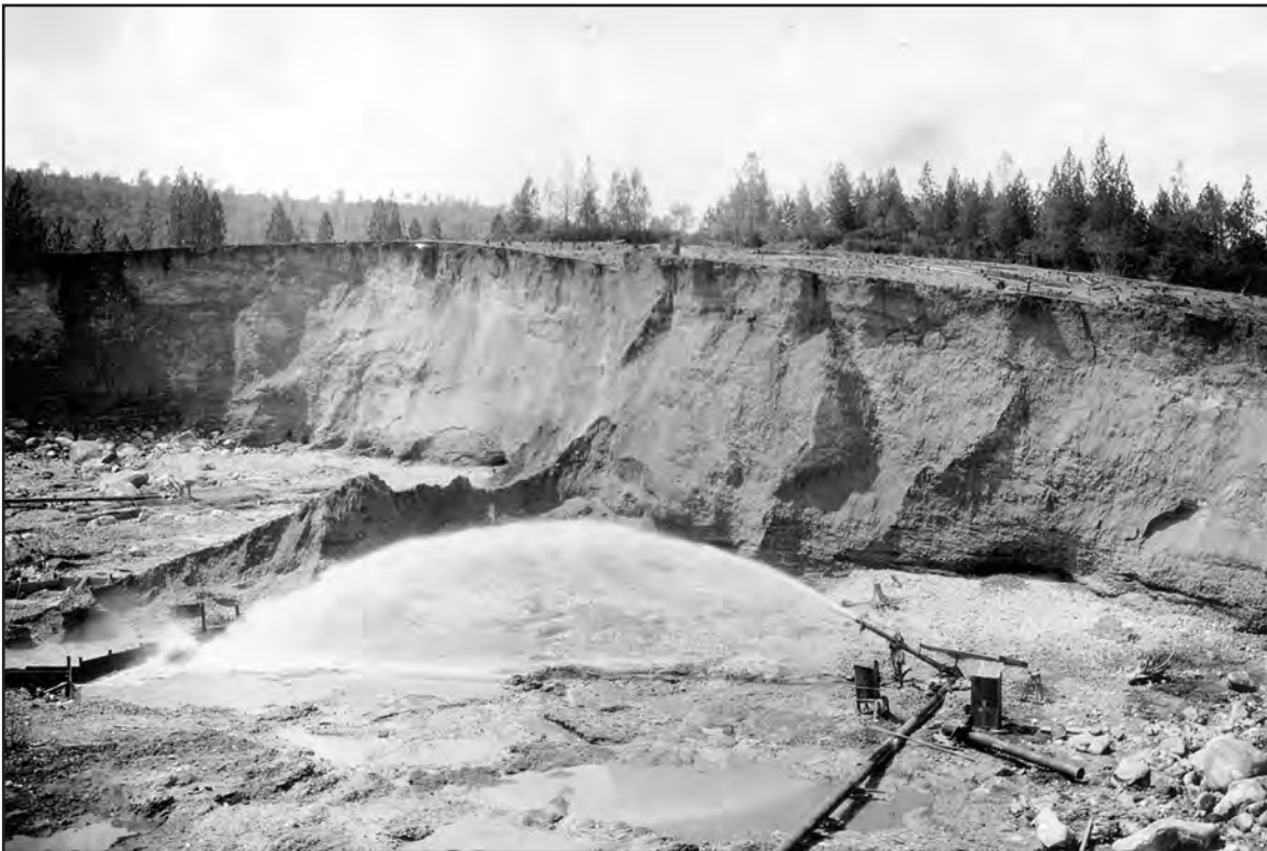
Figure 27. Esperance Hydraulic mine near French Corral, Nevada County, California, 1909. Placer mining for gold removes water from the stream channel. From Gilbert (1917).
