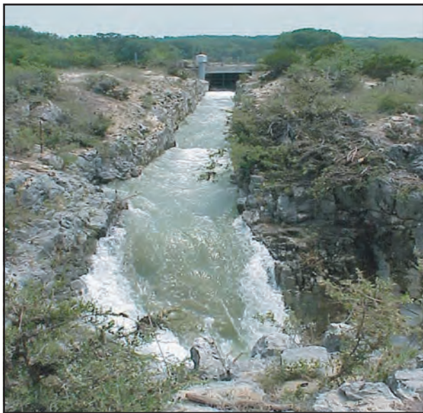
Figure 45. Flood runoff diverted by an engineered channel from Seco Creek to an improved sinkhole that penetrates the Edwards aquifer, Medina County, Texas, July 8, 2002. Photograph provided by San Antonio Water Systems.
