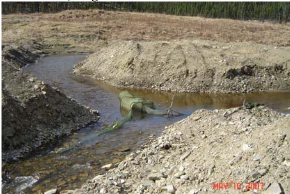
Photograph 5. View of the outlet and constructed island in Pond 1, May 2007.
