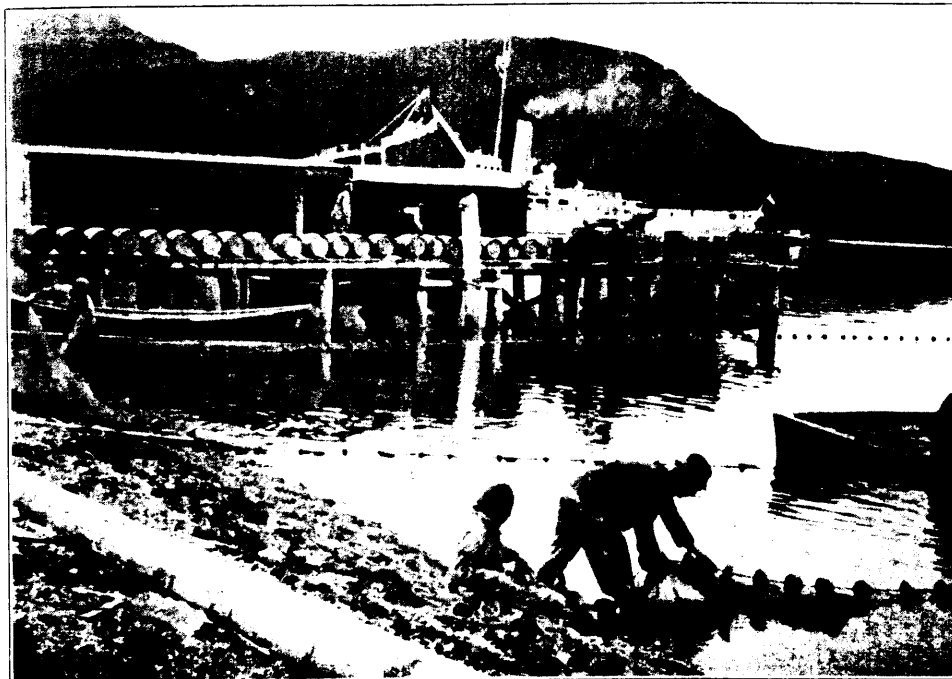
FIGURE 10.—Small saltery erected at Unalaska in 1928. Herring were so plentiful that their pound, consisting of a small beach seine, is right alongside of the dock. The men in the foreground are obtaining herring from the pound for the day's operation
